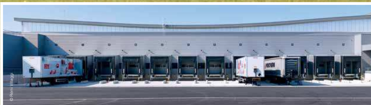
■ Fachada, Danpatherm K7 12 y 16, 900 mm, cristal tratado Softlite, 2.350 m²
